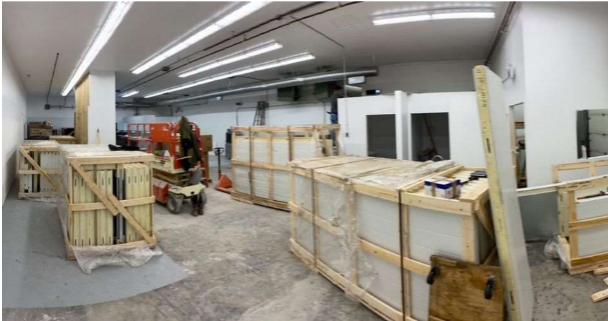
Figure 2 Sprout Kitchen, Quesnel under renovation. Photo courtesy of Sprout Kitchen
